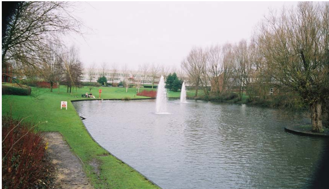
Figure 2: Upper retention pond showing fountains. Willow trees retained and vegetation on the far embankment.
